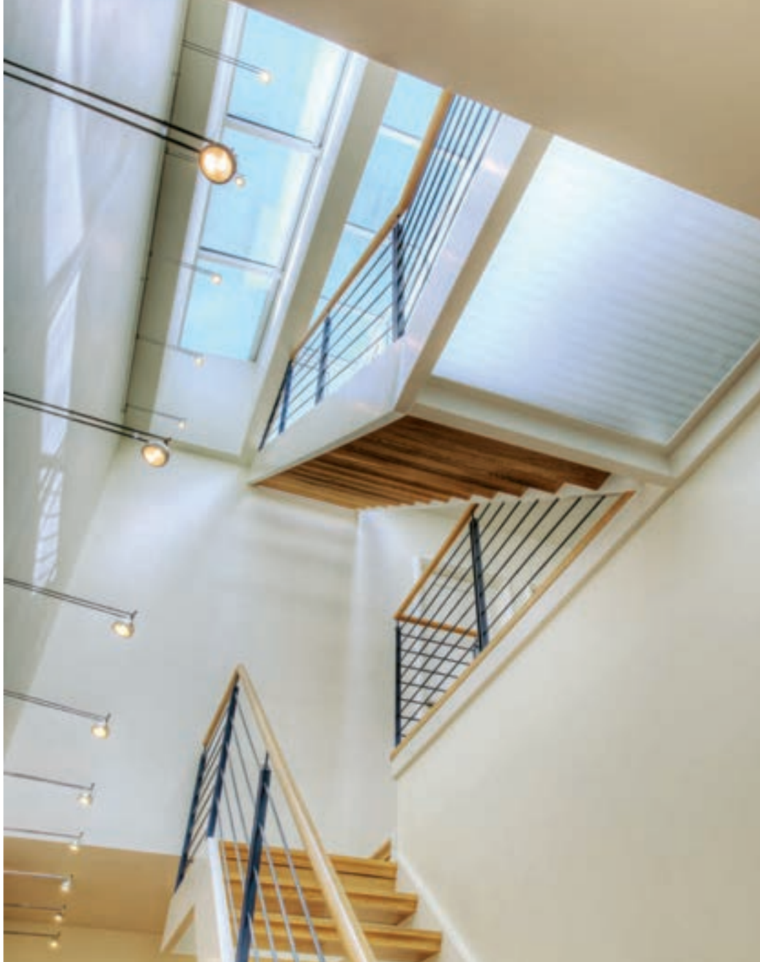
The steel-and-oak stairwell (these pages) spans four flights from the basement to the rooftop terrace. A glass ceiling and opaque glass floor panels flood the house with light, while Monorail fixtures on metal rods from Tech Lighting illuminate the hallways.
